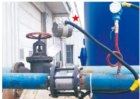
Vortex flowmeter in oxygen measurement
