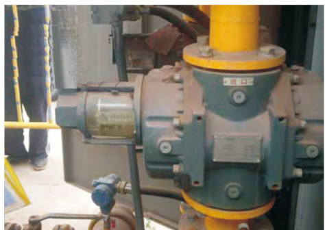
Gas roots flowmeter in gas mixture field
