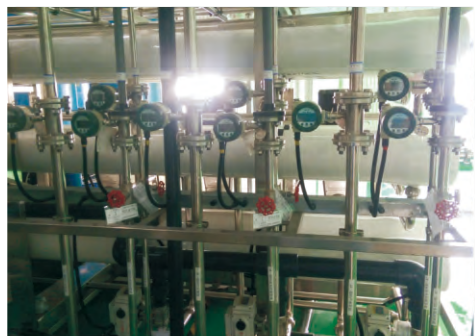
Turbine flowmeter in water supply field
