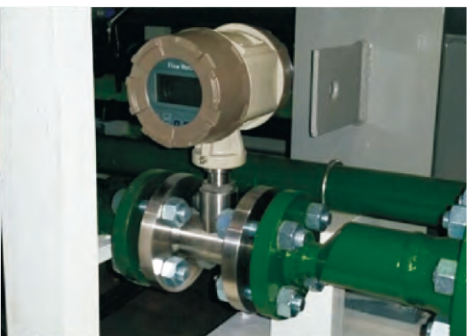
Liquid turbine flowmeter in water supply plant
